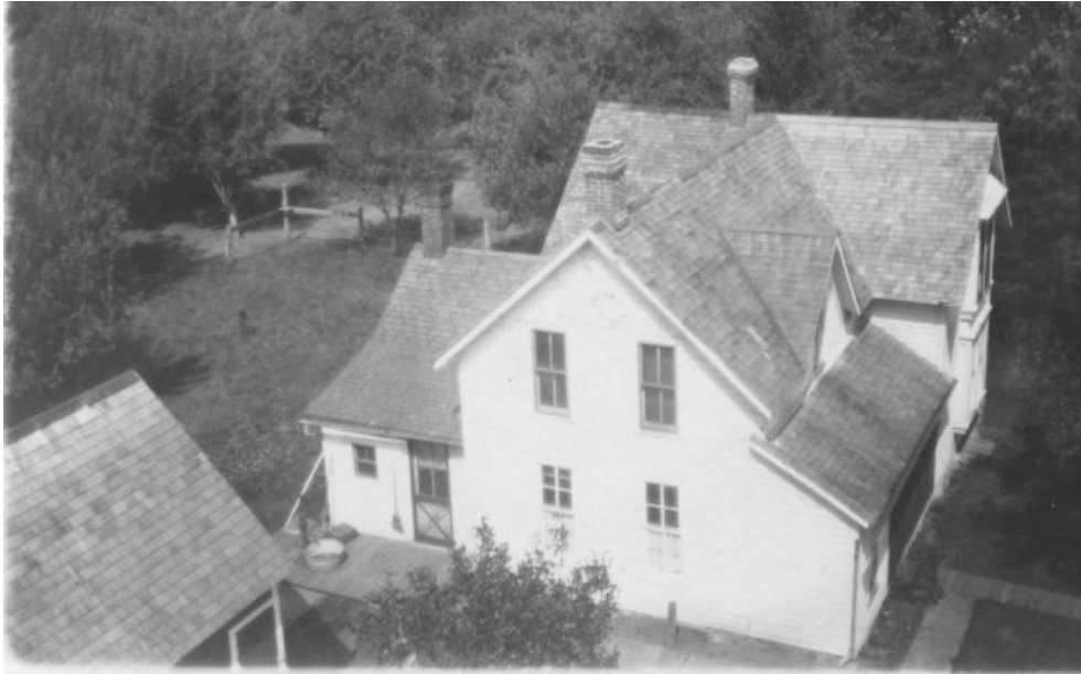
Picture of the house with the old kitchen, cistern pump, and wash house. It was taken from the wind mill.
